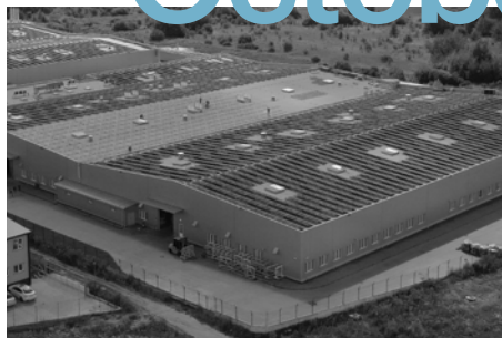
Installation of photovoltaic system in Ukraine
