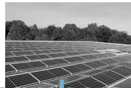
Installation of photovoltaic system in Bulgaria
